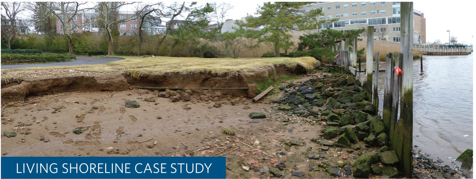
Shoreline at 30 Hubbard Park showing failing wooden bulkhead and severe erosion. © Bill Shadel/TNC
