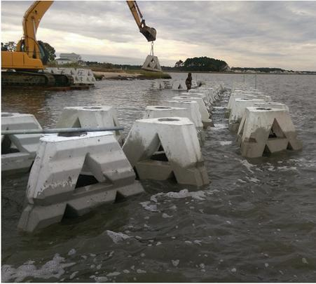
3.5-ft.-high WADs being installed to create a breakwater at the Seagrass Plantation Restoration Site in Delaware © Douglas Janiec
