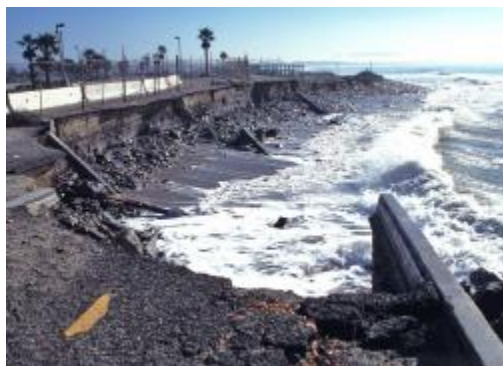
Figure F-7: Project site before (left) and after (right) landward realignment of built infrastructure and restoration of the dunes and beach. The bike path and parking lot were built on fill in 1989 and eroded within 2 years. Photo credit: Paul Jenkin.
