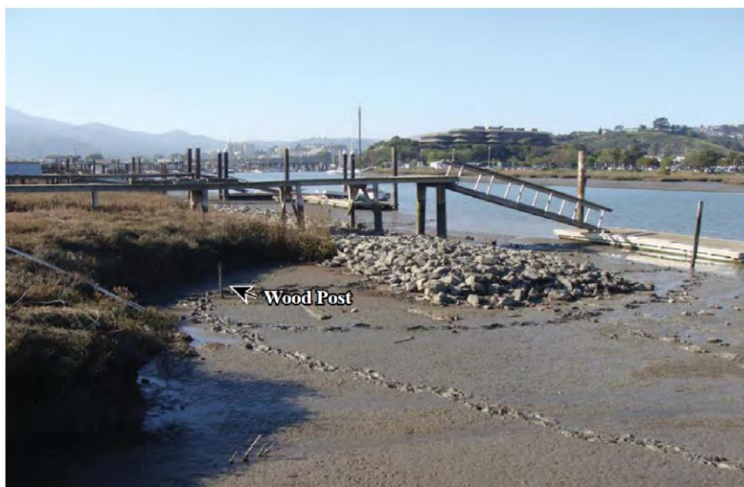
Figure 10. Photograph showing "outflanking", or erosion at the end of a marsh sill, which is typical of coastal structures over their design life (ESA, 2017).
